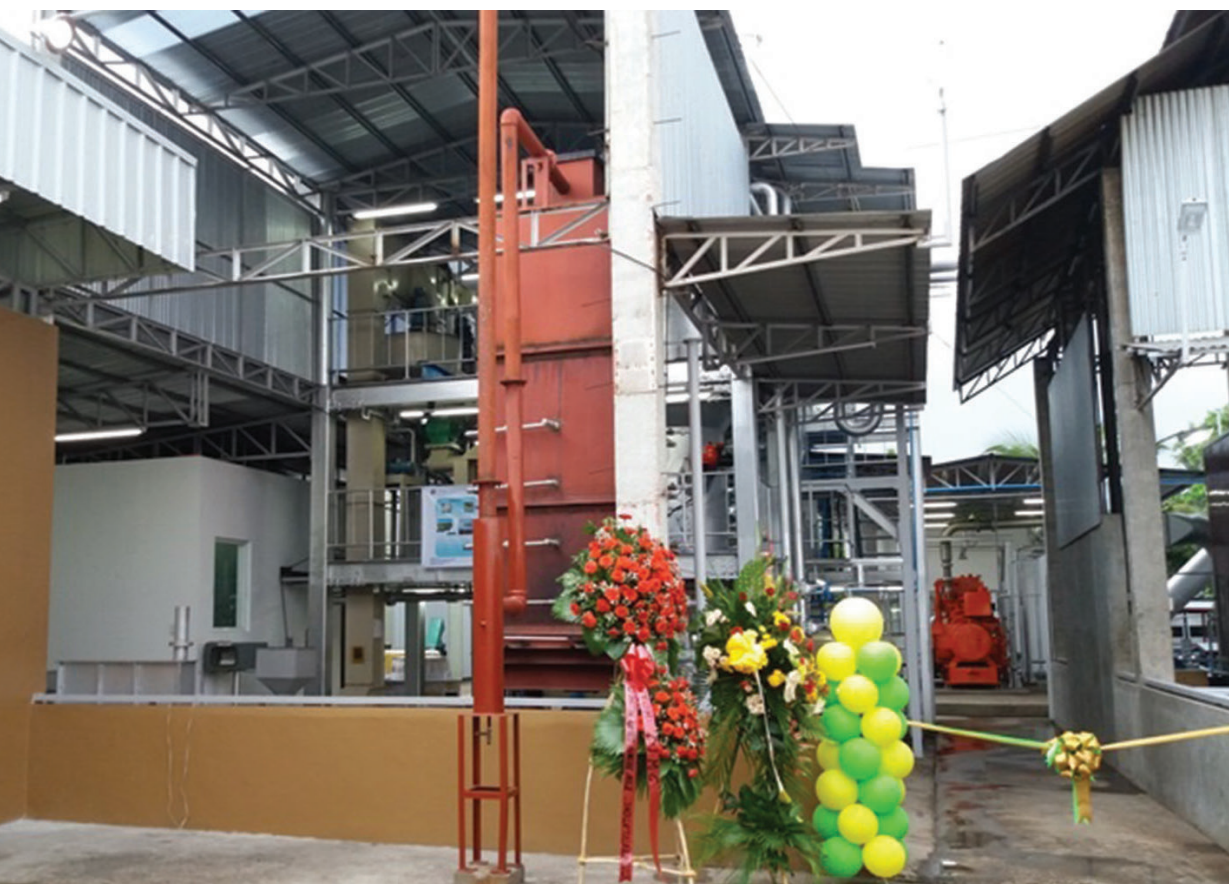
Prototype carbonizer (painted red) is shown in foreground. Behind it is the gasification component (fluidized bed gasifier). (Photo by RBSMCI1)
