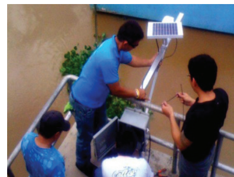
Water sensors being installed in Marikina river
