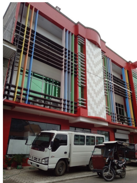
The new cake production facility of Sarah Guarte Cakes and Party Needs in Tandag City. (Photos from DOST-CARAGA)
