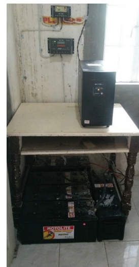
Photos show (clockwise) Rural Health Unit in Brgy. Maniwaya, Sta Cruz, Marinduque is now equipped with a 750-watt Solar Home System. The SHS set-up inside RHU-Bantay with 5 (6sm) batteries, sine wave inverter, and solar controllers. PSTD Bernardo T. Caringal and Mr. Renato Jogno oriented and demonstrated to Dr. Rowena Grace Garcia the newly installed Solar Home System in RHU-Bantay.
